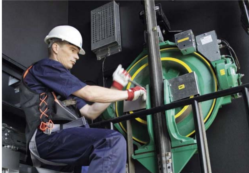
Figure 2.8. Kone axial flux permanent magnet machine for gearless elevators [Kone 2013].
