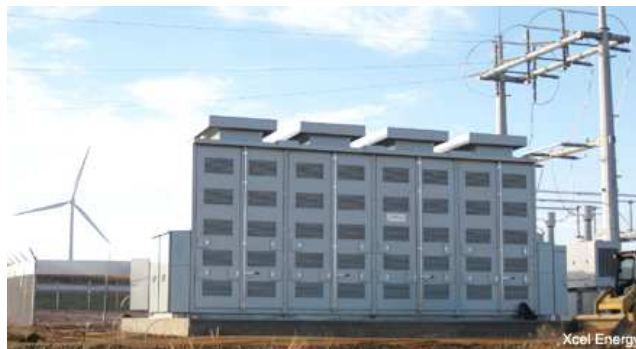
Figure 11: NaS battery module
