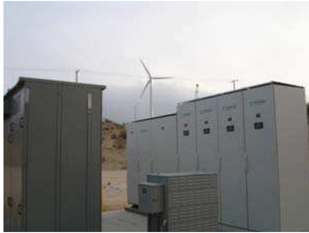
Figure 15: Ultracaps Energy Storage System, Palmdale, California, USA
