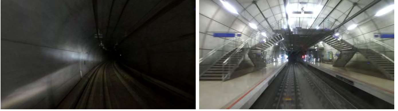
FIGURE 1: The CAF dataset's tunnel and platform areas where the poor light conditions and textureless areas can be appreciated.
