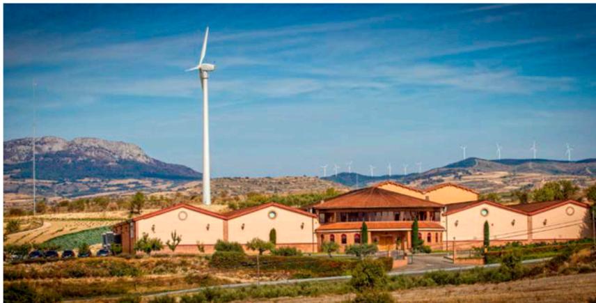
Figure 1. Wind Turbine of 100 kW placed in Bodegas Pierola wine cellar (Moreda, Araba, Spain).
