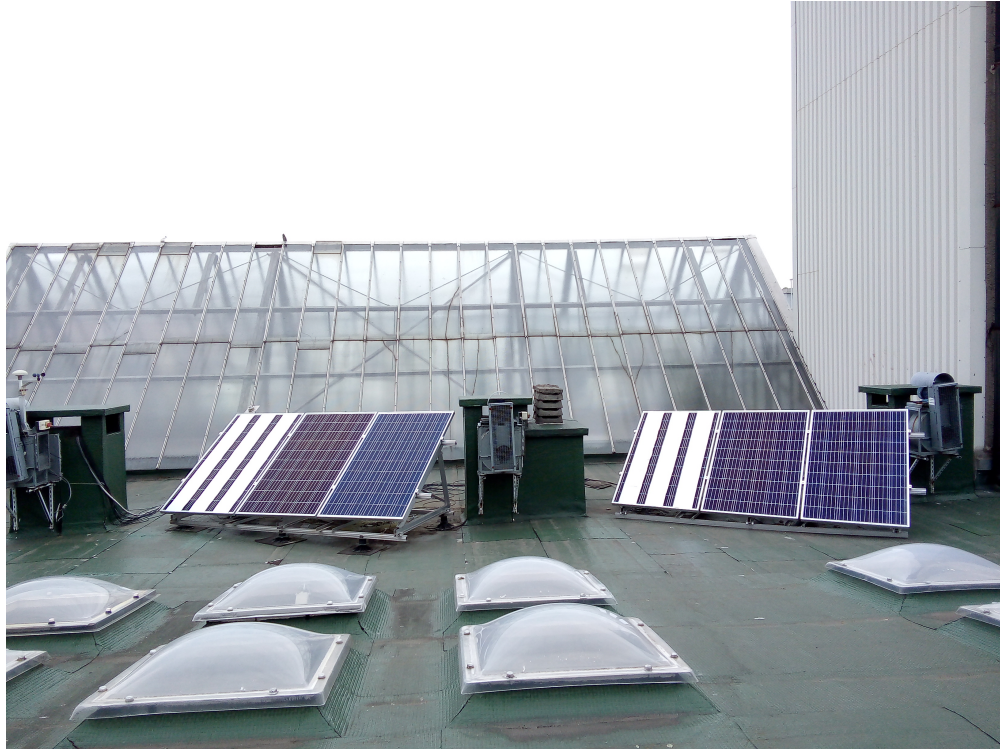
FIGURE 9.6: PV1 to PV6 from left to right - Sh \simeq 50\% static shade on PV1 and PV4.
