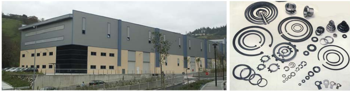
Figure 3.1: a) Outside view of Industrias Alzuaran S.L. located in Zaldibar (Spain) and b) Family of parts produced at Industrias Alzuaran S.L.
