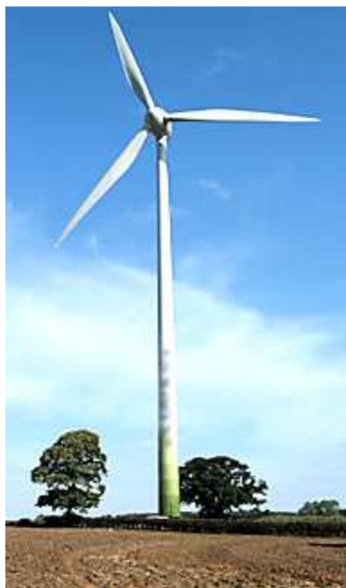
Figure 2-9: Commercial wind turbine with horizontal axis.
